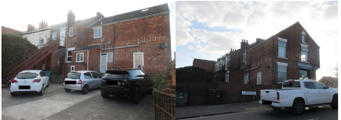
Side and rear elevations of application site
